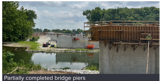
Partially completed bridge piers
